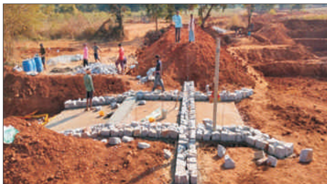
Construction of outlet of the farm pond at Tara village
