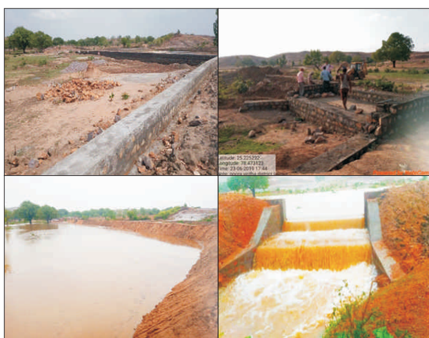
Fig. 43: Haveli structure from excavating foundation to various construction stages in Birdha village of Lalitpur district; Structure received good amount of runoff from the upstream hillock
