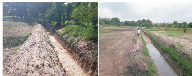
Fig. 45: Diversion drain for safe disposal of excess runoff from uplands to stream network; top two pictures from Birdha village, Lalitpur; bottom pictures from Sutta/singar village, Jhansi
