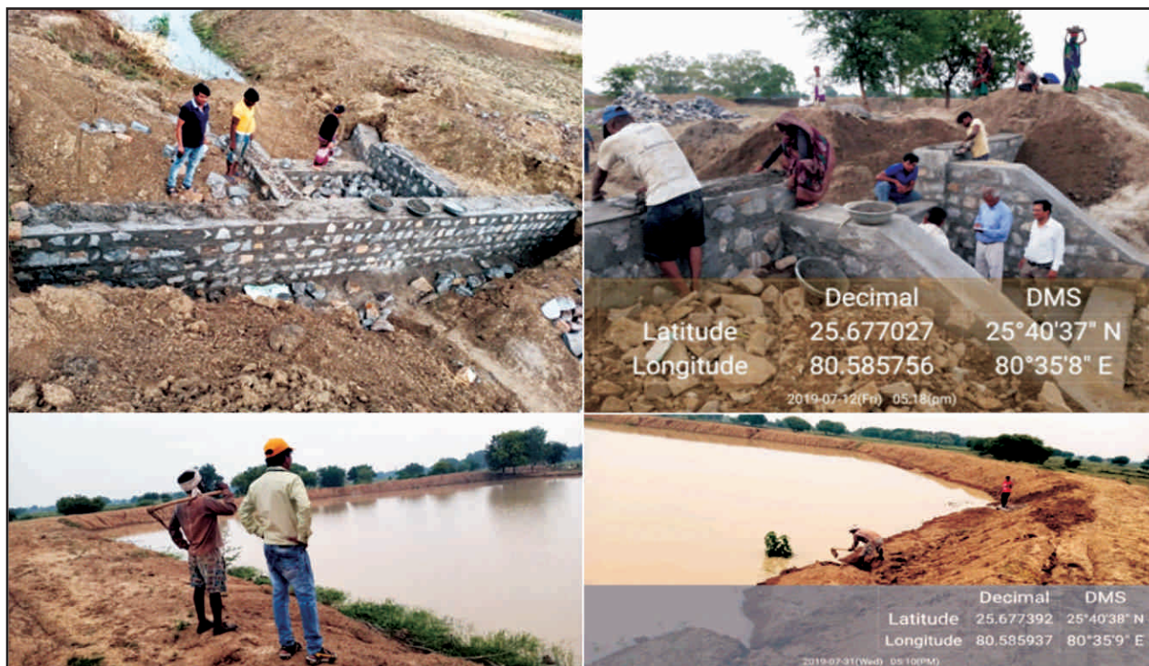
Plate 24d: Village tank which is renovated in Banda; Nearly one 1.5 ha area desilted and masonry outlet was constructed for safe dispose-off the excess runoff
