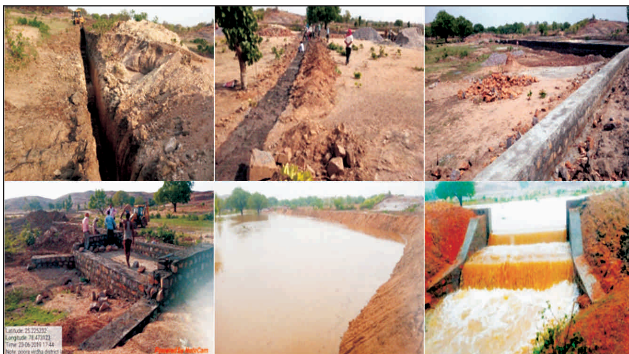
Plate 24c: Haveli structure from excavating foundation to various construction stage in Birdha village of Lalitpur district; Structure received good amount of runoff from upstream hillock
