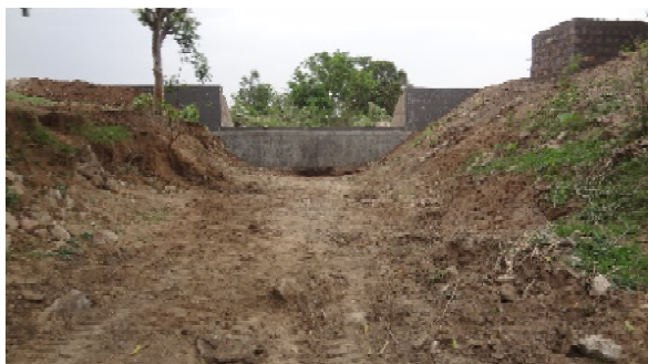
Drop structure and gauging station in Bachhauni village of Watershed
